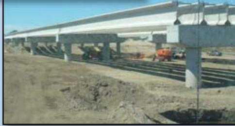
As part of the Twin Peaks interchange project, partially funded by the RTA, the Town of Marana and ADOT, 60 concrete bridge girders were delivered in early September for the bridge going over the Santa Cruz River. Each girder is 120 feet long.
